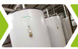
Incoming water is pre-heated using the waste water reducing energy consumption across the entire site
