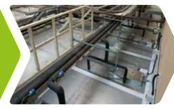
Waste heat from the refrigeration is syphoned off to a heat exchange
