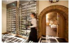
The Towers are all 3 metres high by 1.5 wide. Two have glass sides all round and three have stainless steel backs, to go against the wall. Four are connected to remote refrigeration, whilst the fifth uses its integral system.
