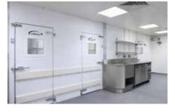
There are seven chilled coldrooms (+1/+4°C) and one freezer room (-18/-22°C), plus a prep room at 10°C, as well as another room for beer in the basement. Williams coldrooms feature a modular construction and a range of panel sizes and colours that allow designers to create bespoke rooms to virtually any size or shape.
